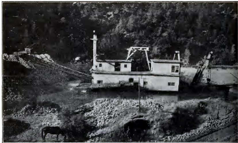
Photo No. 30. Bucyrus Dredger of the Pacific Gold Dredging Co., working near Mammoth Bar on the Middle Fork of the American River.
