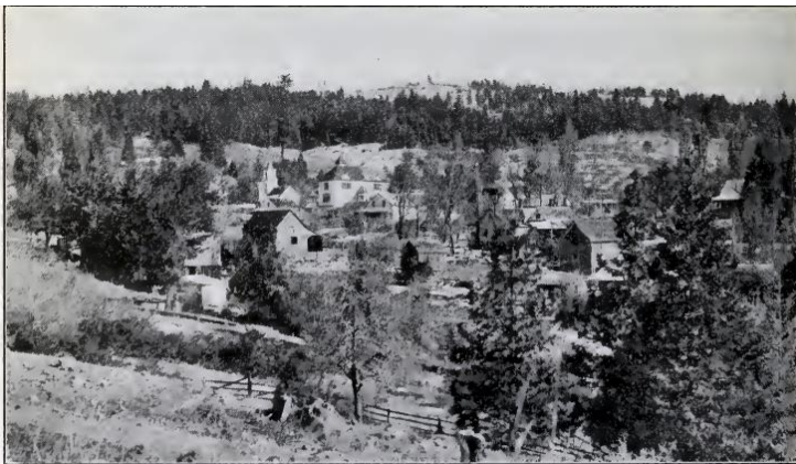
Photo No. 12. View eastward towards the town of Dutch Flat. The X in center marks the location of the Federal Drift shaft.
