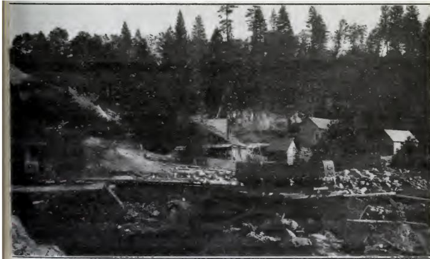
Photo No. 18. View eastward of the Pacific Slab Mine, Last Chance District, showing office, cook house, gravel bin and hydraulic monitor.
