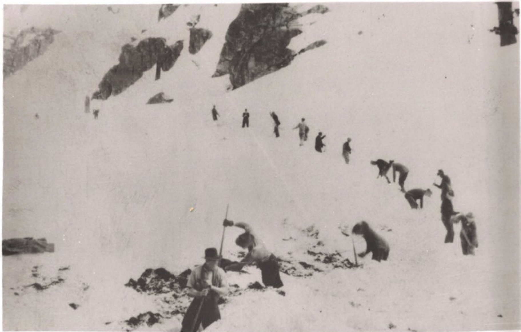
Digging Out Donner Summit 1930
